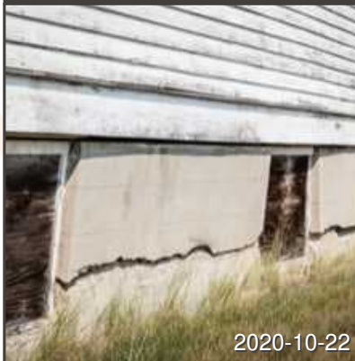
Damage to foundation
