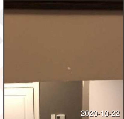
Damage to drywall on stairs
